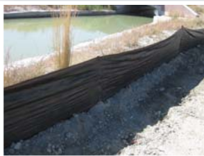
Silt Fences (Biologs may be used when the ground is frozen)
